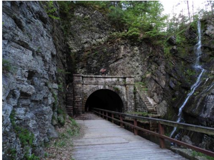
I am standing on the top of the Paw Paw Tunnel Exit. Deceptively long at 3118ft.
