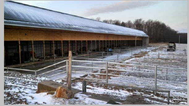
Great progress rebuilding from the fires
